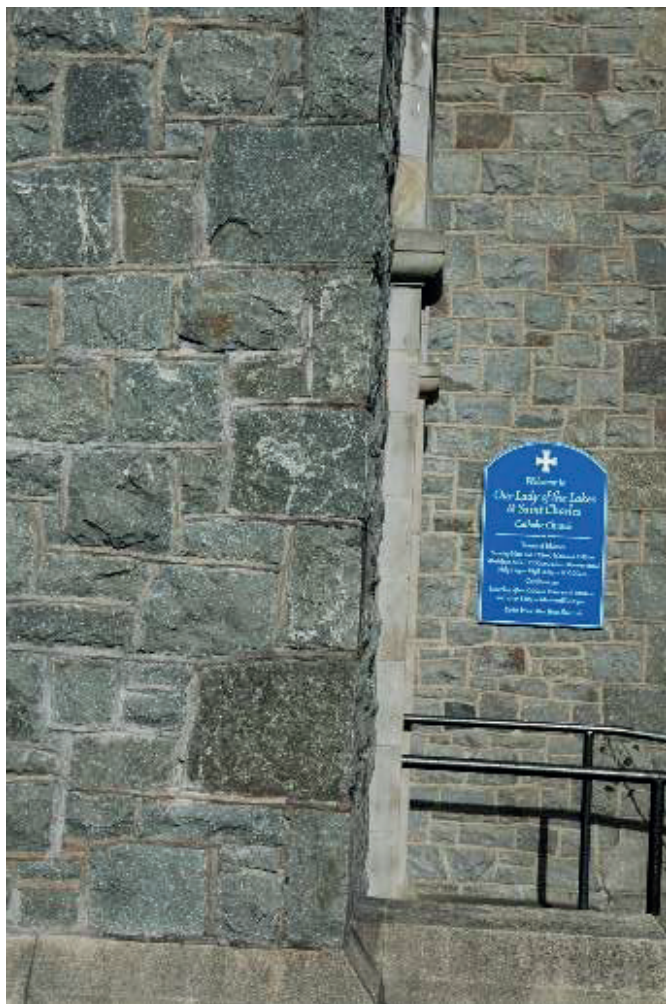
Picture 3. Our Lady of the Lakes and St Charles Church showing detail of the Threlkeld Microgranite walling material.
