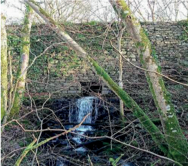
Cuddy Beck culvert underneath the A591 at Lonsties
