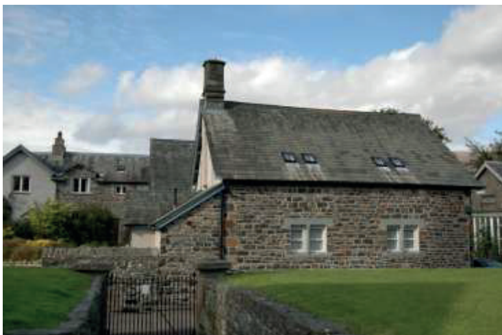
Picture 6. The former St John's School, St John's Street. Walling of Castlehead Diorite and roofing in Lakeland Greenslate with graduated coursing.
