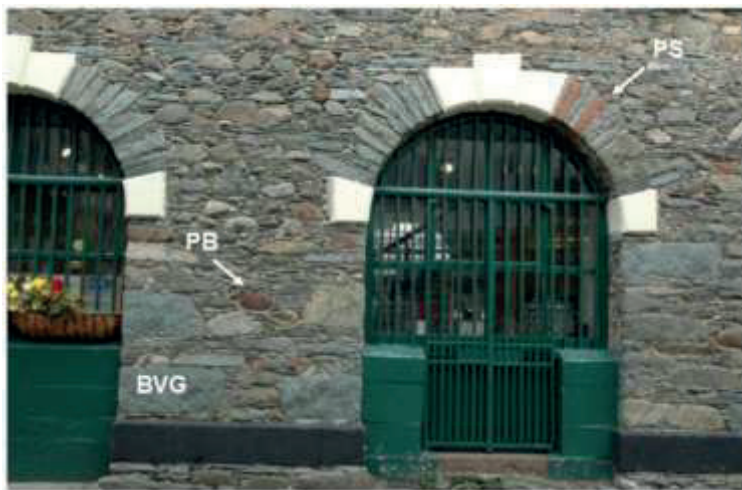
Picture 1. Side wall of the Moot Hall BVG - Borrowdale Volcanic tuff on edge PB - Purple Breccia PS - Penrith Sandstone
