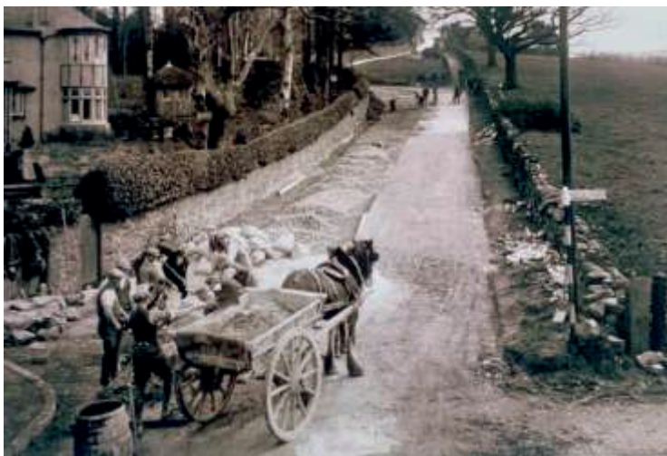
1920s roadworks on Manor Brow. Only Borrowdale is decipherable on the guidepost that is pointing down Springs Road.
