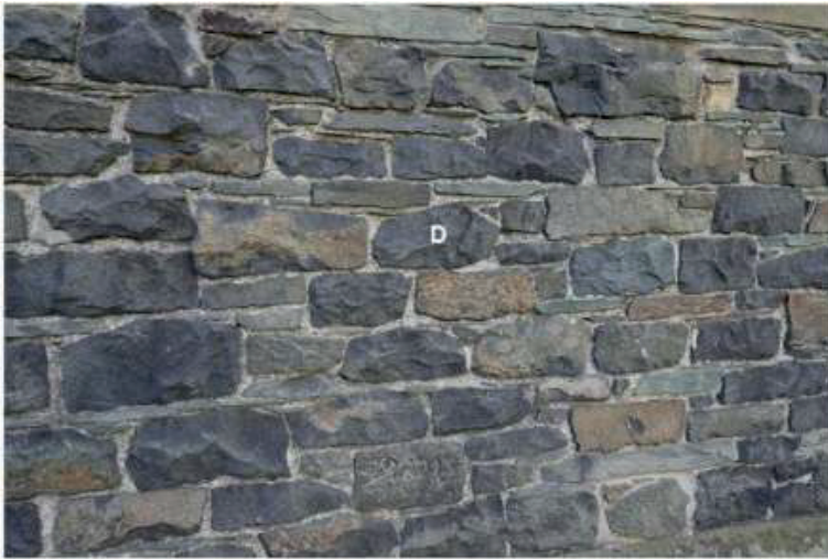
Picture 5. Wall of St John's School D - Section across a hexagonal column of diorite
